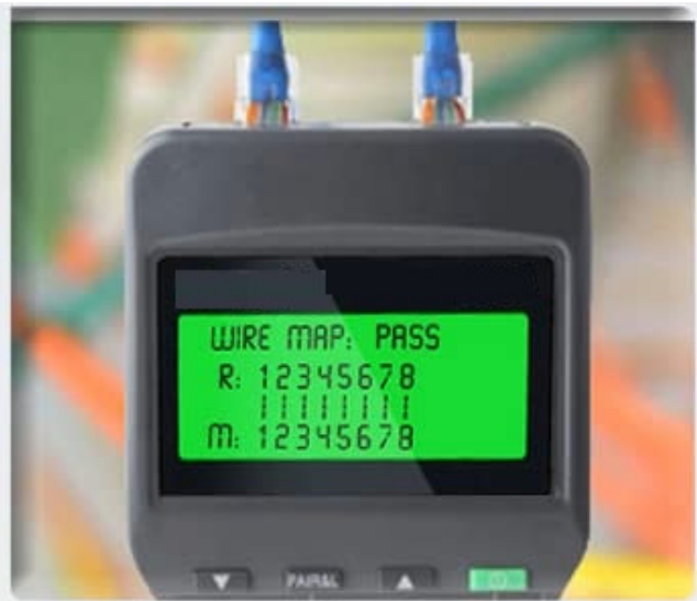
Cable Continuity Testing
